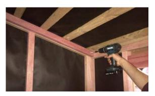
Step 15: Using 2 x 75mm framing nails, nail centre roof purlin to front and back top plate stiffeners. Predrill if necessary.
